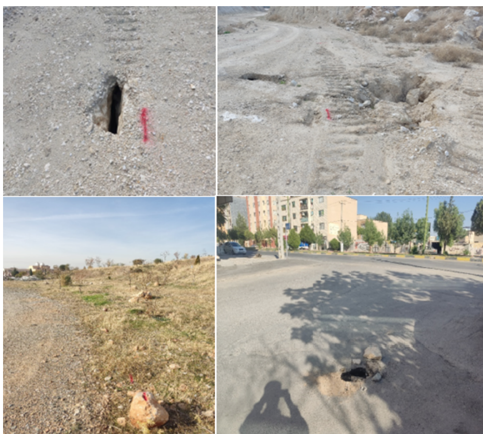
Figure 5. Image of the study areas: The road under construction (upper), the asphalt-covered road with cavities (lower right), and the road on a small old tunnel (lower left)
